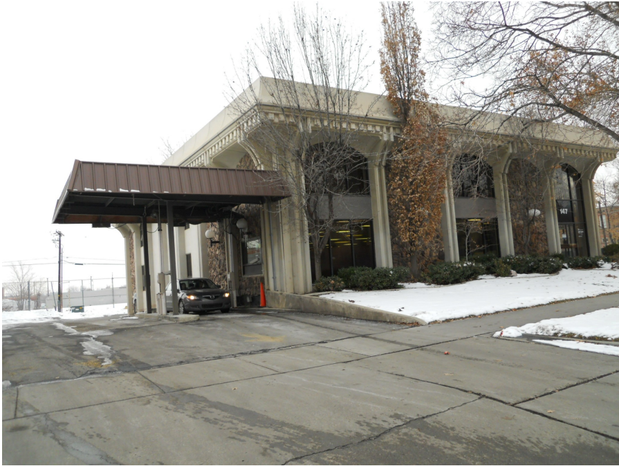
South Entrance and drive-through to be removed
